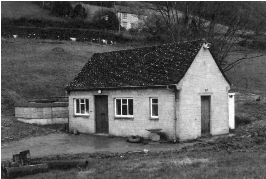
Fig. 9 Millend pumping station (North Nibley)
