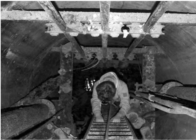
Fig. 4 Dursley Well pumping station (1902). Descending the well
