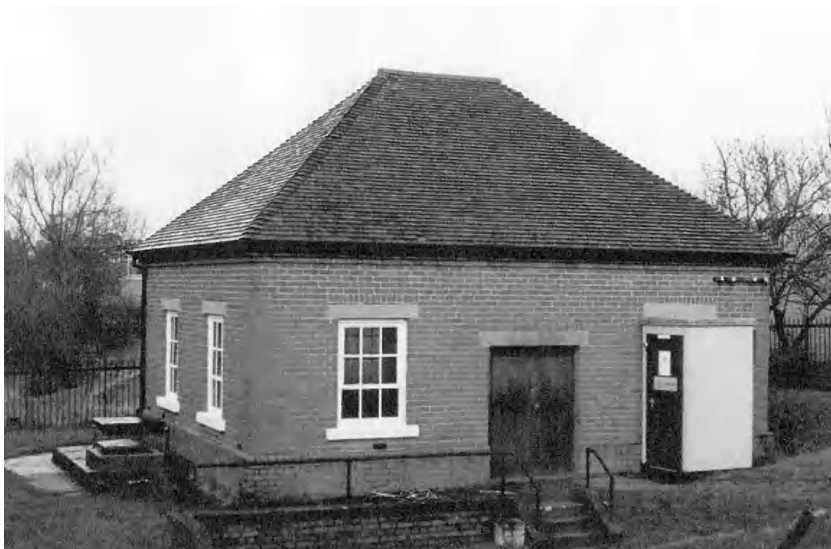
Fig. 7 Dursley (Caswell) pumping station. After completion in 1935
