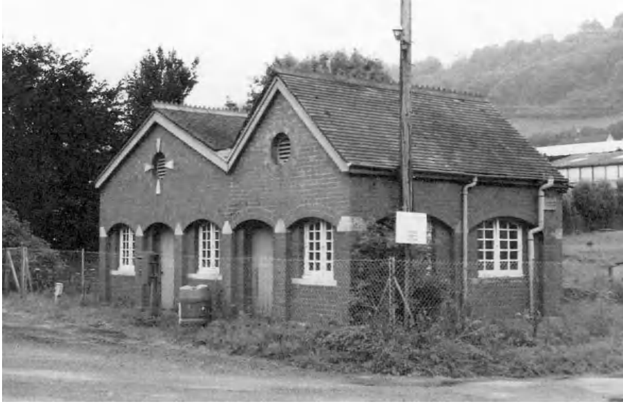
Fig. 10 Coombe pumping station (Wotton-under-Edge). Opened 1909
