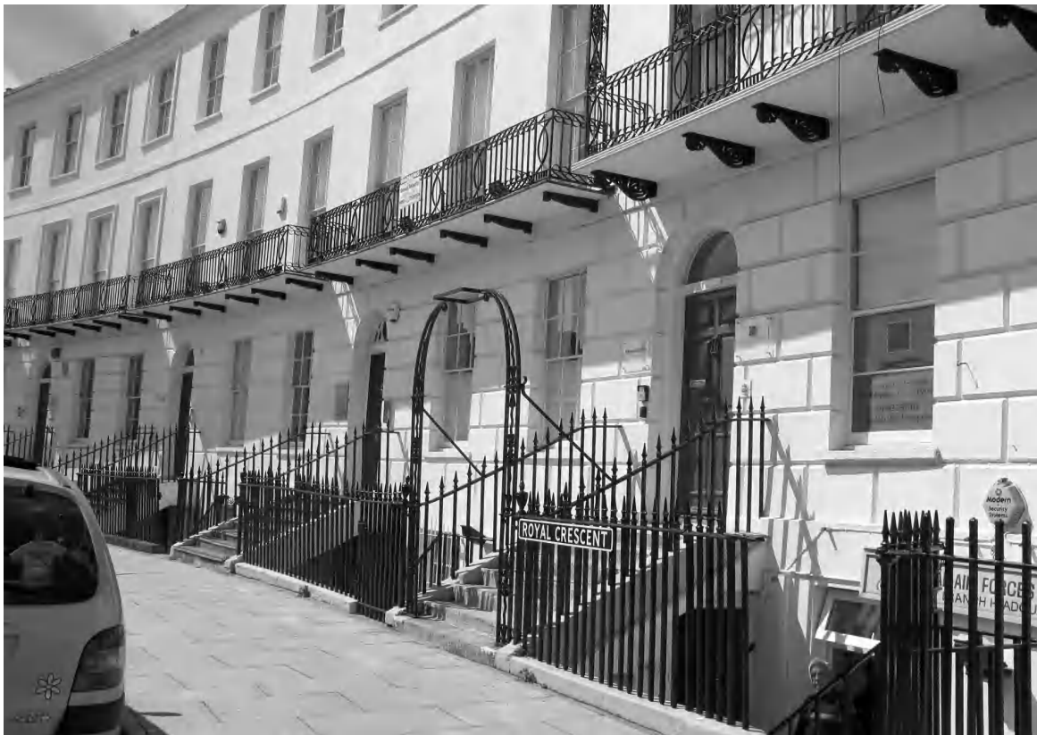
Ornamental Ironwork in Royal Crescent, Cheltenham. Sunday 24 July 2012
