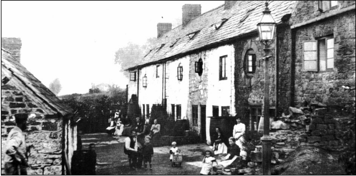
Photograph from c. 1902 of Factory Cottages Looking South (4)
