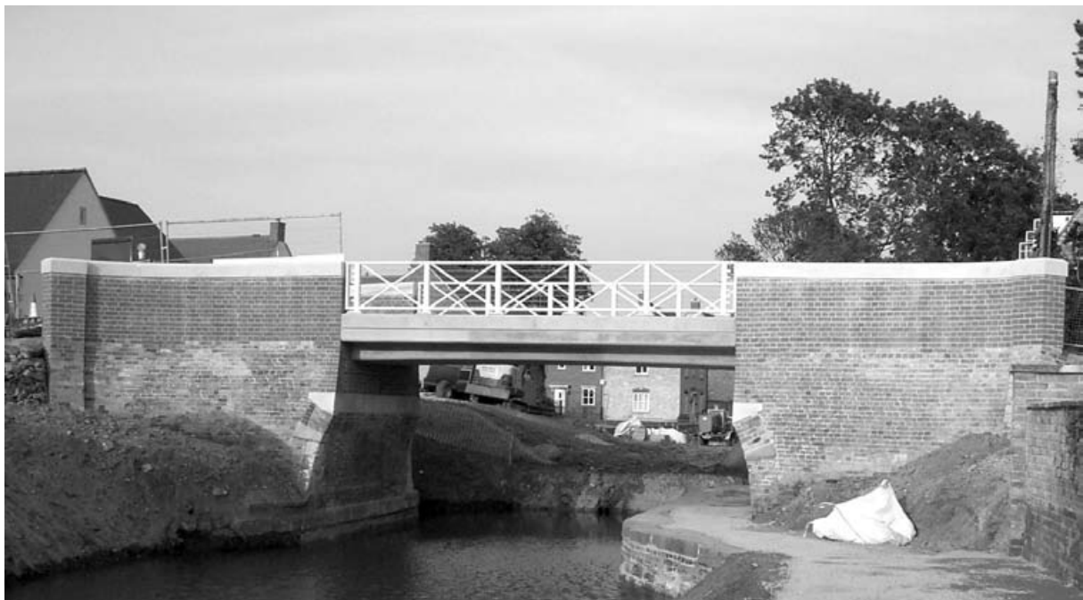
The new Oil Mills bridge nearing completion in May 2008, looking east.
