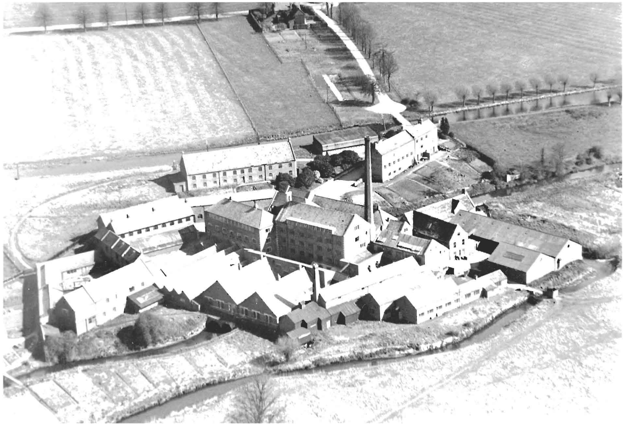
Fig. 3 Bonds Mill, Stonehouse, c1930. The close proximity of the Stroudwater Canal is clear
