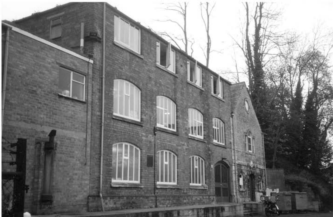
Figure 6. Former offices and warehouse (on right) at Wallbridge Mill seen from the east in 2005.
