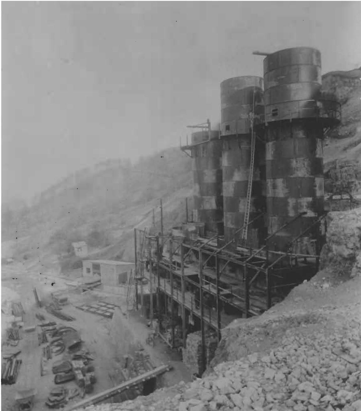
Plate 1      The Focal Point of the Railways (C2) in 1924 Showing the Four Limekilns (D1) Under Construction (looking north-east).
