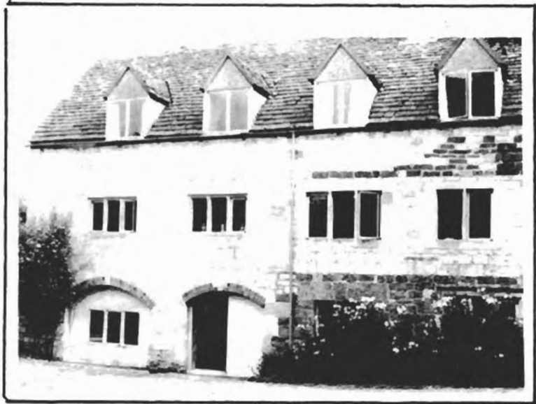
Damsell's Mill from garden side. Inside the doorway an over-shot water-wheel is preserved.
