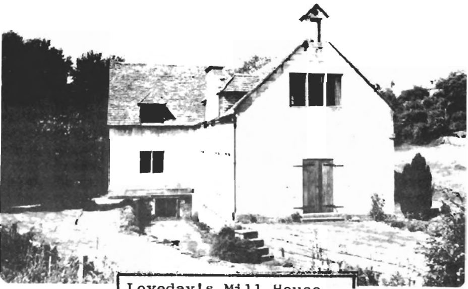
Loveday's Mill House (note bdlfry & site of mill leat to left)
