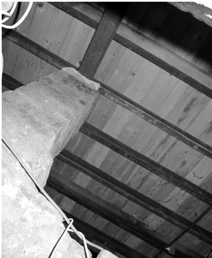
Malt kiln at Chipping Campden malthouse showing the stone bearers on which the tiles are laid. The tiles on the right hand side of the picture are ready to be laid. Note that their bearers are supported on bigger stones at right angles which in turn are supported by stone and some cases brick pillars.
