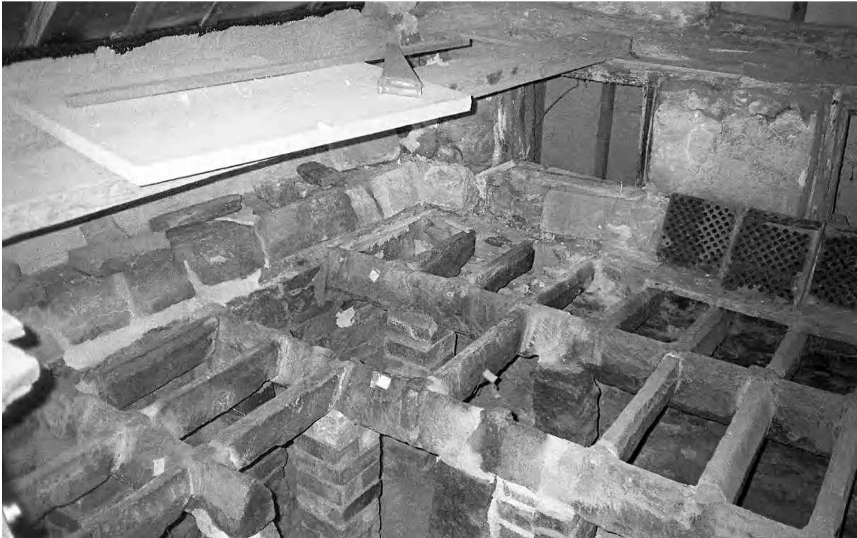
Malt kiln at Chipping Campden malthouse showing the stone bearers on which the tiles are laid. The tiles on the right hand side of the picture are ready to be laid. Note that their bearers are supported on bigger stones at right angles which in turn are supported by stone and some cases brick pillars.
