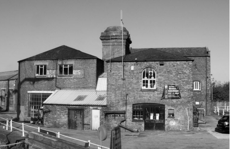
Fig 5. Engine house viewed from the east
