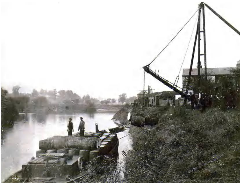
Tar barge Kathleen with barrels on the deck and a barrel being transferred by the derrick crane.
