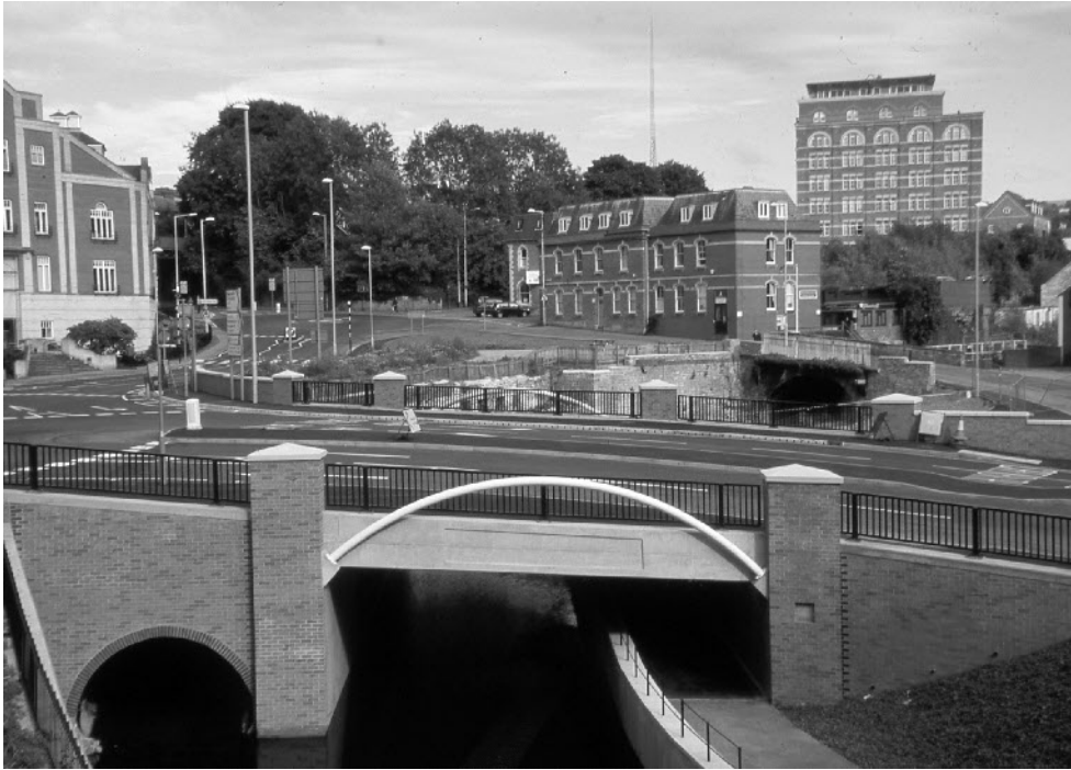
Figure 2 The new Stroud Brewery Bridge looking east
