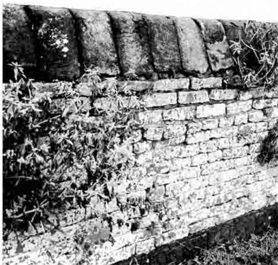
Figure 9. Triangular copper slag blocks used as wall copings at Nastend House, Nastend, Eastington,
