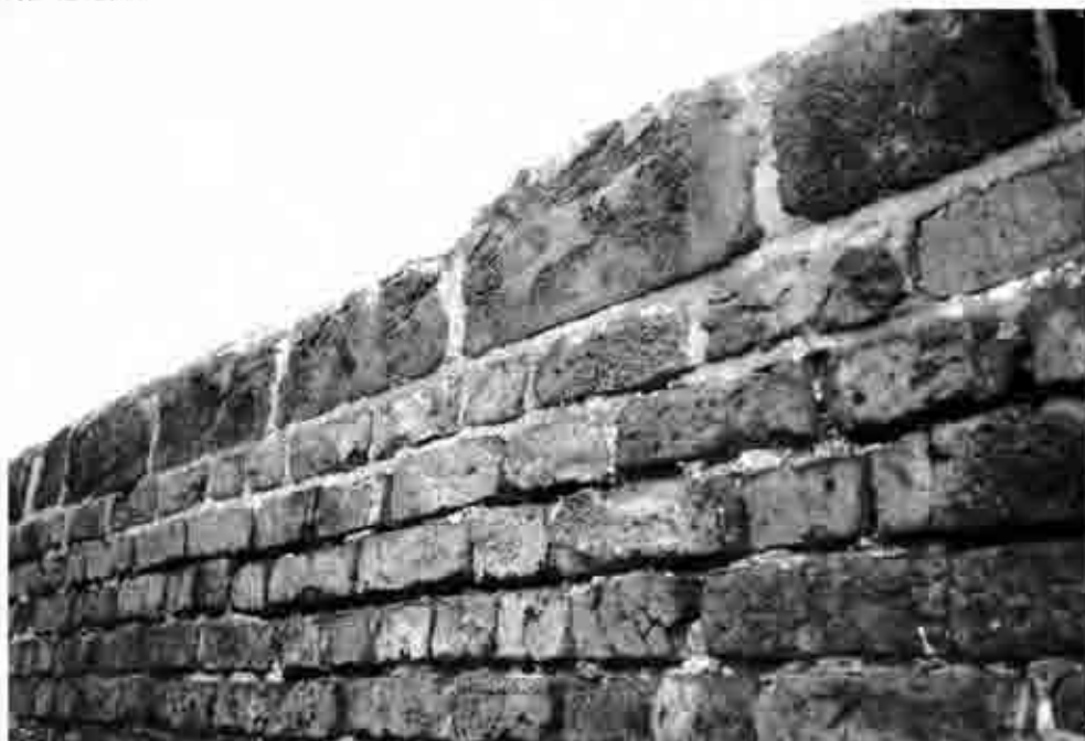
Figure 1. Rectangular copper slag blocks used as copings on a wall beside Organ's Alley, Gloucester
