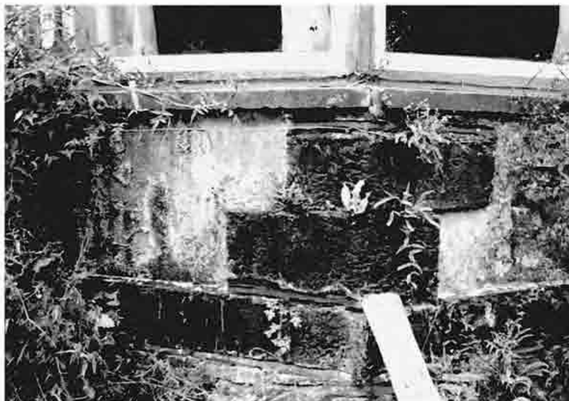
Figure 12. Angle-ended, bay type rectangular copper slag blocks at Highbury Farm, Redbrook, Newland
