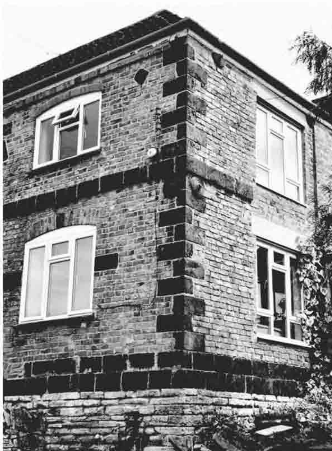
Figure 7. Use made of slag blocks at Corner House Farm, Corse
