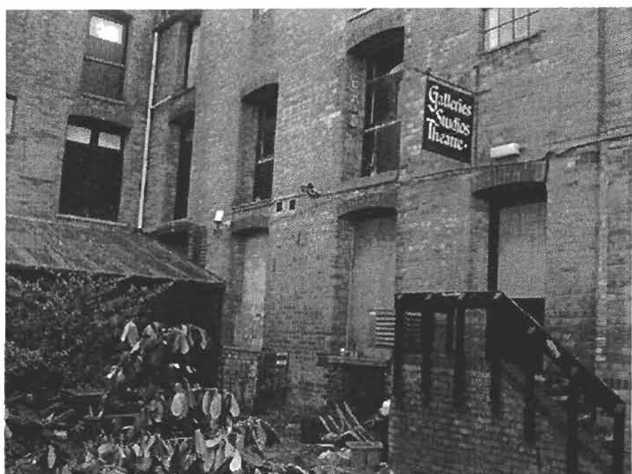
Figure 2. 57-59 Winchcombe Street (North-east elevation)
