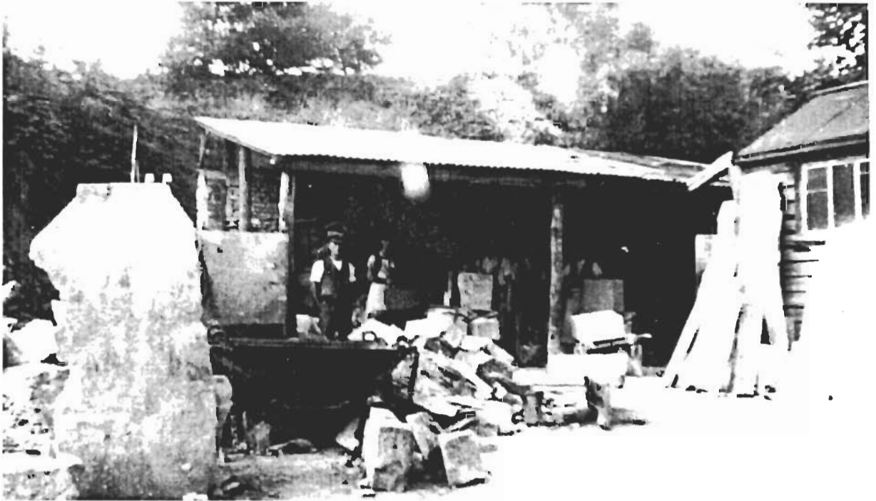
The sawing and banker mason's shed at Tuffleys Quarry.
