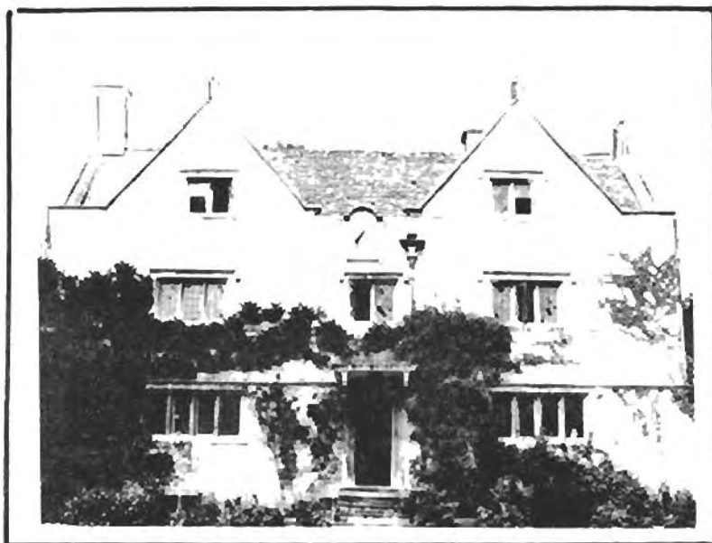
Tocknell's Court: clothier's house connected with Tocknell's Mill of which nothing at all now remains.
