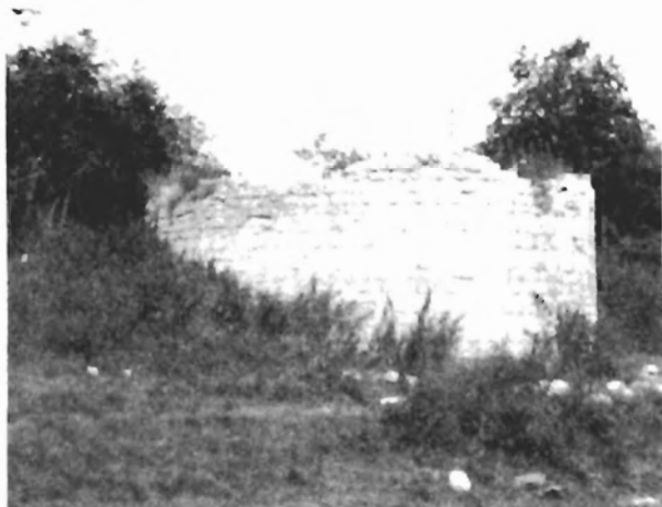
The remains of the Wool Drying Stove at Upper Baylis' Mill. The bank of the former millpond can be seen in front of the ruins.
