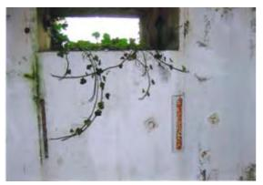
Ref 3.7 G Mountings for support shelves below embrasures FW3/26 pillbox showing remains of metal angle bracket screwed to timber fixing which has been cast into the wall Site CCD
