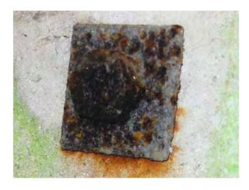
Ref 3.7 B Rusting of panel retaining bolts Site CCD
